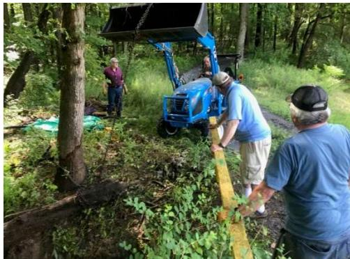
With Bill Leaman at the tractor's wheel, the team secured a chain around tree trunk and successfully pulled it out of the feeder stream unclogging the culvert and reestablished the water flow. With the tree trunk and debris removed, the stream should flow as intended keeping the road around the lake intact.
