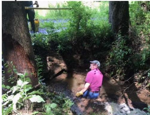
Jay Copsey volunteered to climb into the overflowing feeder stream where the water was chest high and began clearing the culvert opening with the help of Tom Vegella, Bill Jackson and Bill Leaman. The team was able to remove most of the debris with the exception of a large fallen tree trunk.
