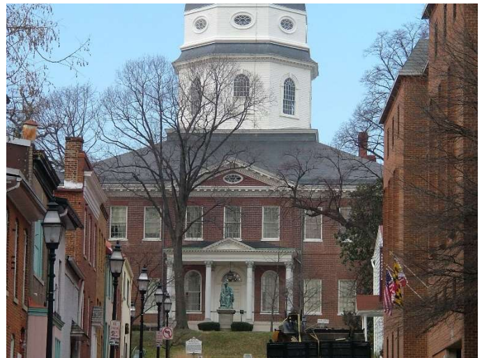
Maryland Capitol Building
